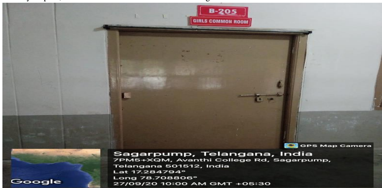
Women Waiting Room at First Floor, EEE building
